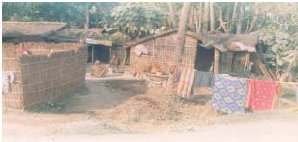
A view of the rehabilitated huts in village Purnahi on 22 nd September, 2003. (Bihar)
