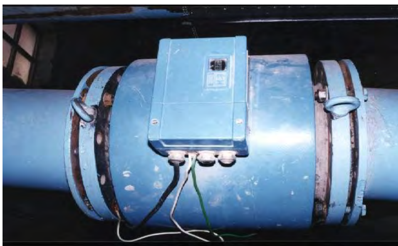
Photo 3-2: The electromagnetic flowmeter
