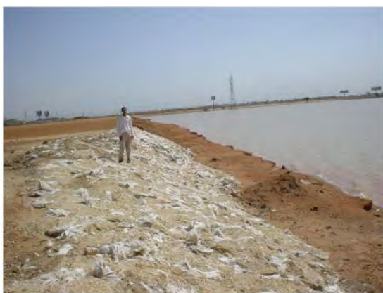
Figure 5-7: White Nile eroded bank
