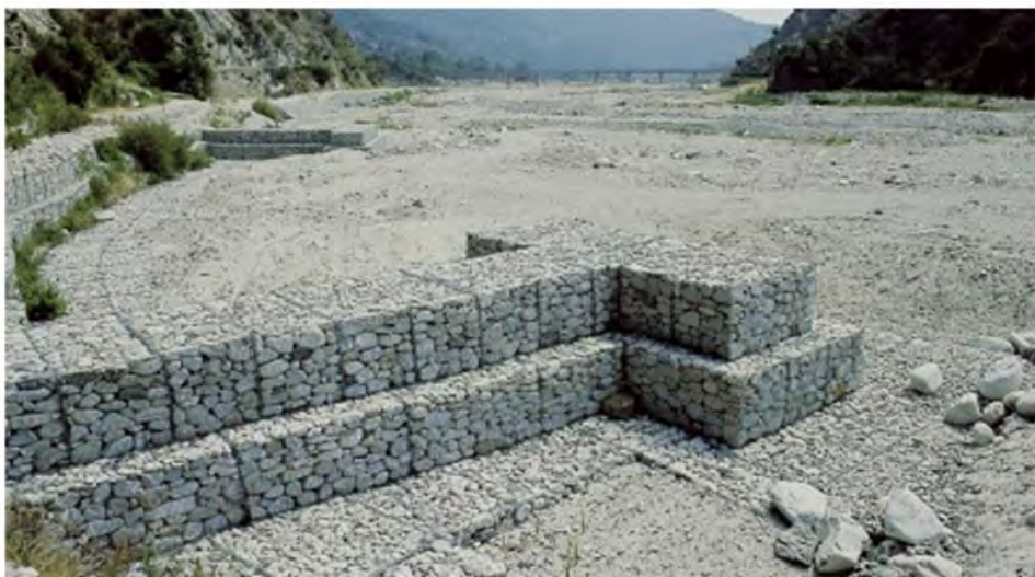
Figure 5-15: Typical gabion groynes in construction
