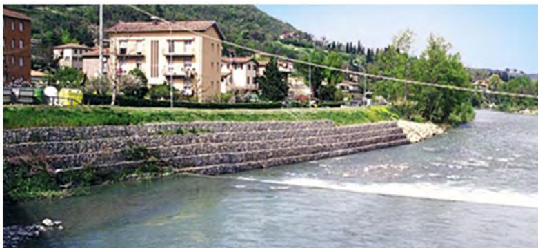
Figure 5-14: Typical guide bank gabion walls
