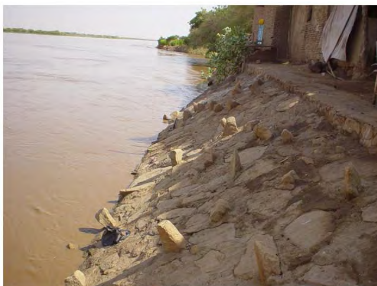
Figure 5-9: Main Nile eroded and protected banks
