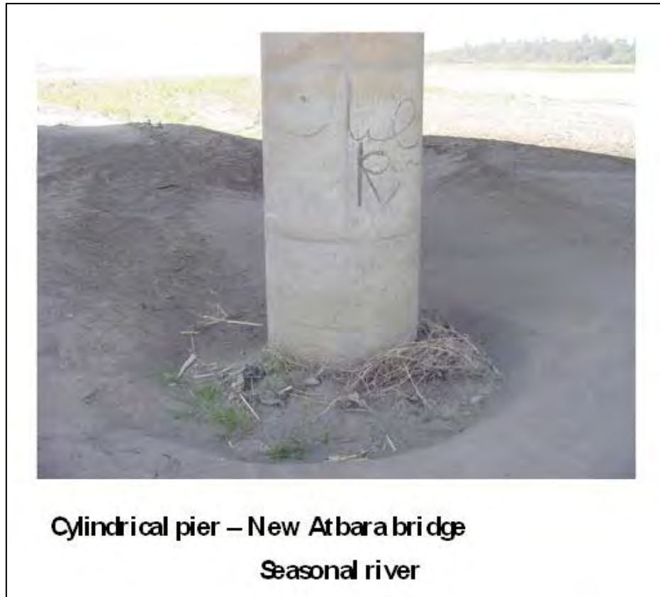
Figure 6-17: Live bed scour in the Nile River
