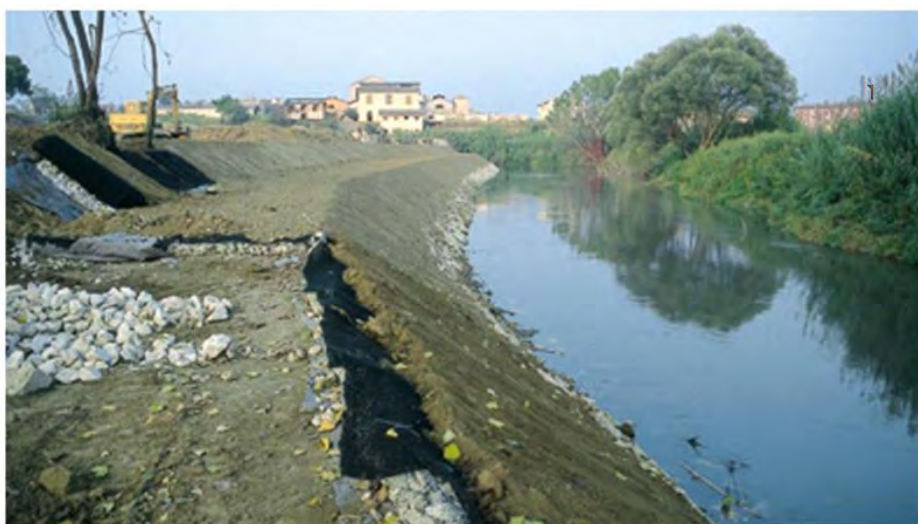
Figure 5-16: Guide bank failure
