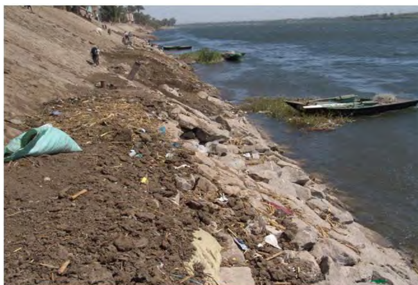
Figure 6-2: General view of bank toe protection
