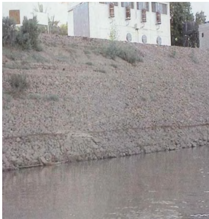
Figure 3- 8: Protection of pumping station at El-Gaba –Northern State by rock and cement
