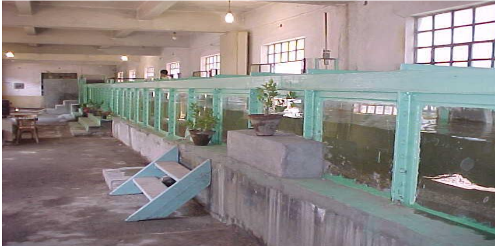
Photo 3-1: General view of the flume
